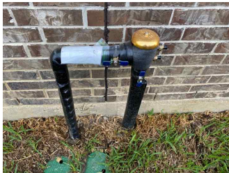
View of the the sprinkler system backflow prevention device
