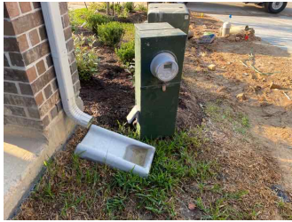
View of the meter and main breaker panel
