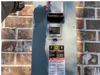
View of the main breaker panel
